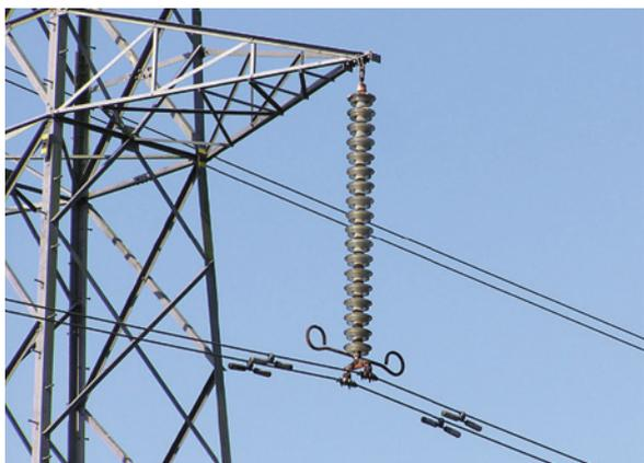
Insulators are useful for separating electricity from objects and living things that it could damage. In the picture at the left, power lines are separated from the metal tower by a stack of ceramic insulators.
